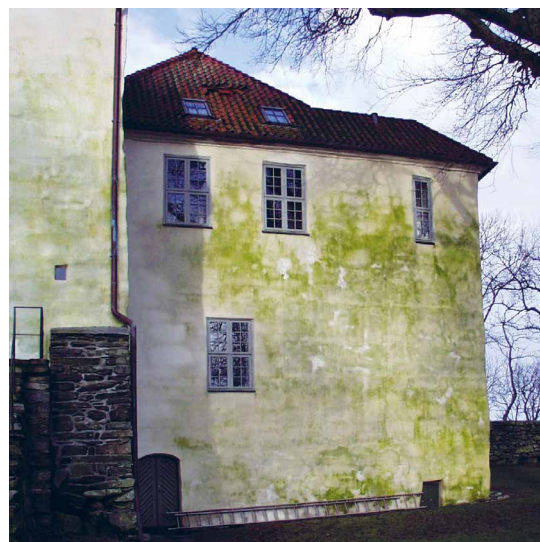
↑ INCREASED BIOLOGICAL GROWTH on building facades is a growing problem due to Increased humidity and rainfall. Utstein Monastery, Stavanger Municipality. Photo: Johan Matsson, Mycoteam
