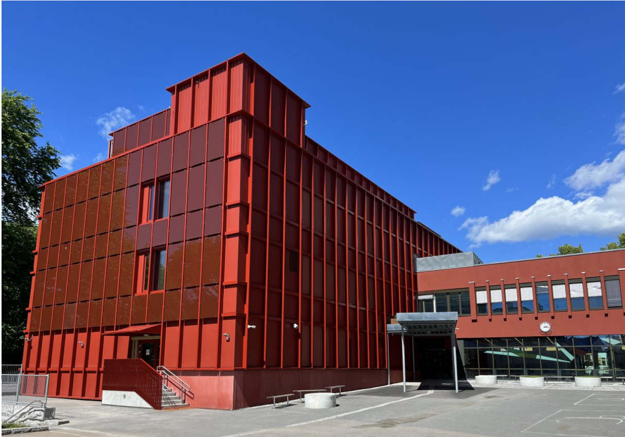
The building has been completely refurbished and has solar panels on both the roof and the facade. Photo: Cato Mørk, Multiconsult
