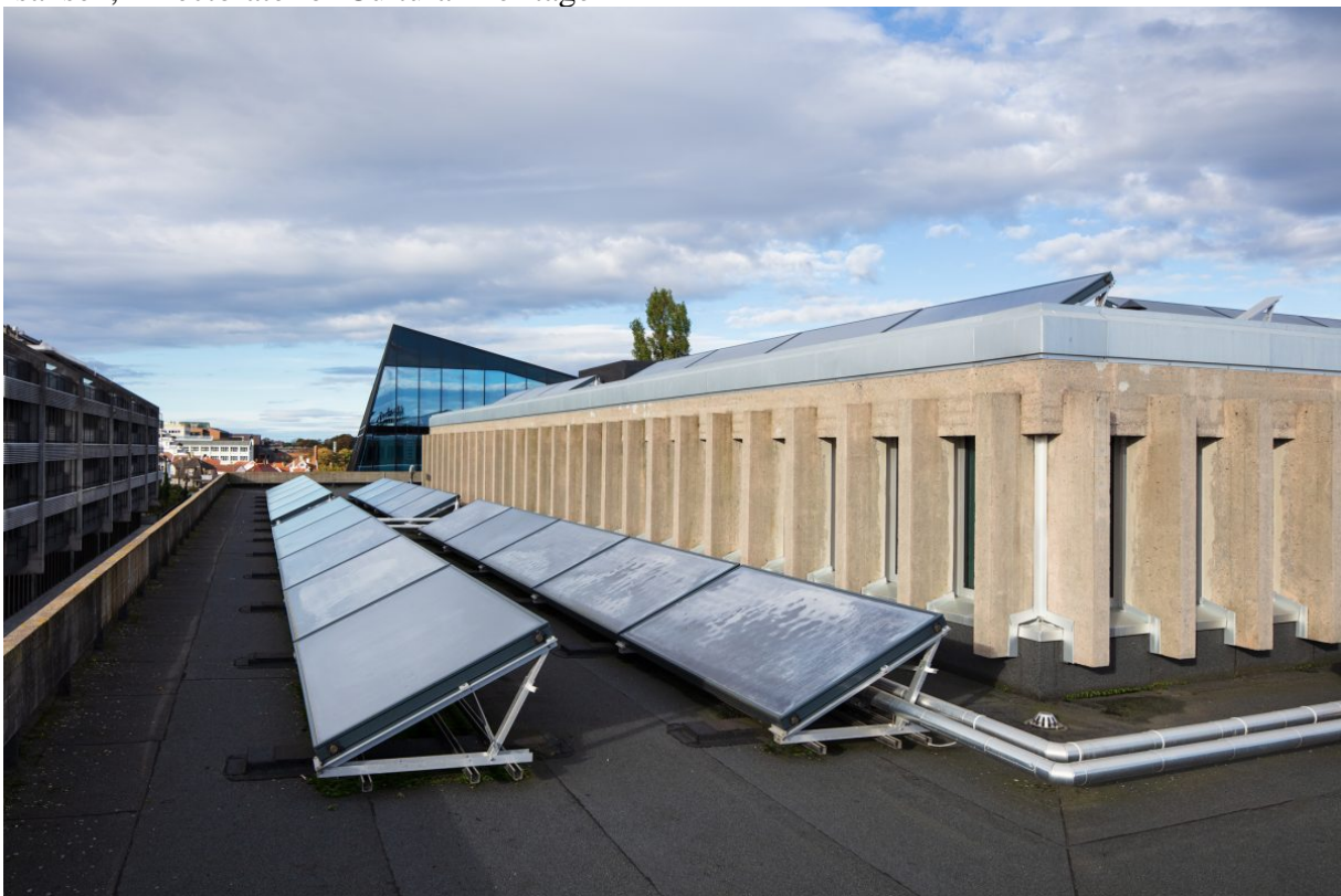
Following input from the Cultural Heritage Management Office in Stavanger, the solar collector system was reduced in size and moved further away from the edge of the roof so that it is not visible from street level. Photo: Trond Isaksen, Directorate for Cultural Heritage
