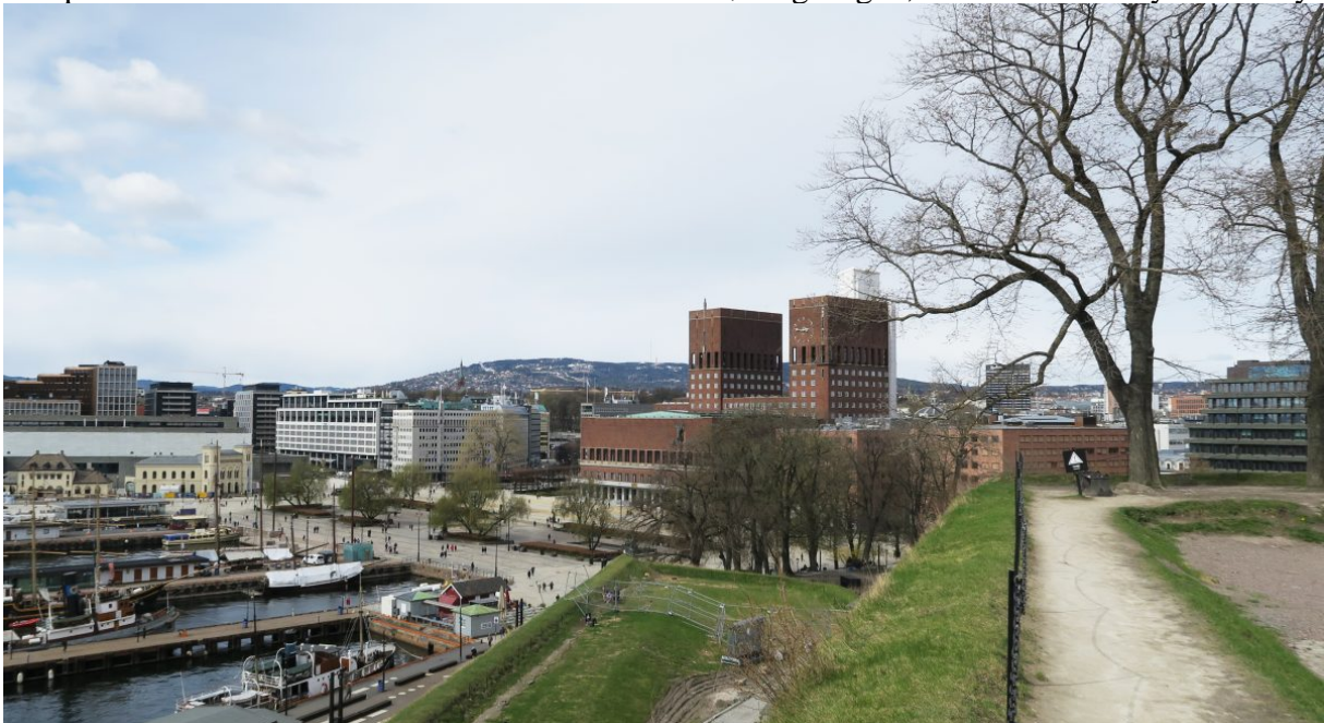
Oslo City Hall has installed a photovoltaic system on parts of the roof. The photovoltaic system is visible from the towers, but not from public spaces or the ground below. If one looks very closely, they can just be made out from the top of Akershus Castle. Photo: Karen Elkjær, Directorate for Cultural Heritage
