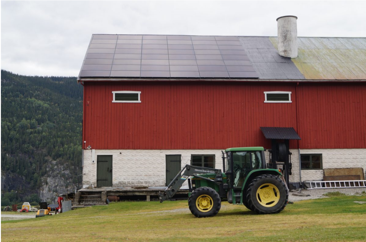
At Elstad Farm in Ringeby, solar panels have been installed on parts of the farm building. The colour and framing of the panels are well adapted to the corrugated iron roofing, and the panels are systematised in a good way. The panels cover one entire area so that they do not compete with the roof surface below. Photo: Tore Røbergshagen, Innlandet County Authority
