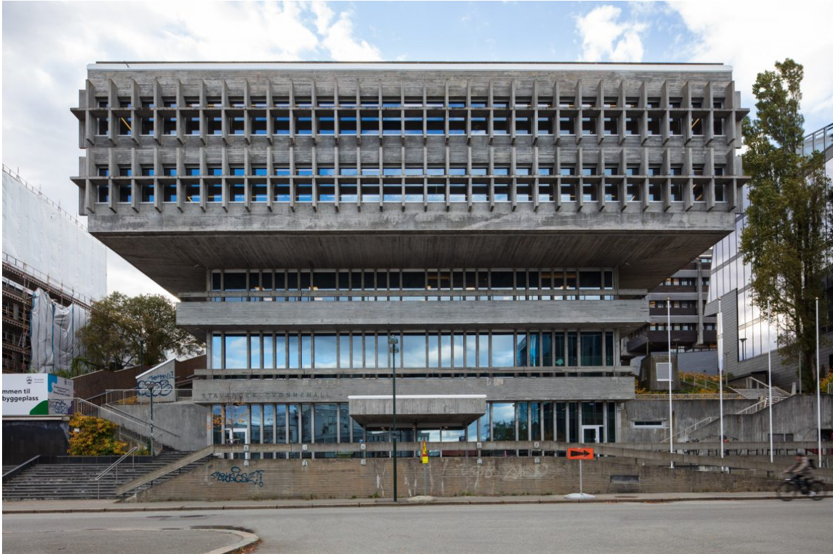
Stavanger Swimming Pool is a brutalist style building from 1971, designed by Gert Walter Thuesen and Jacob Grytten. It has now had solar collectors installed on the roof. Photo: Trond Isaksen, Directorate for Cultural Heritage
