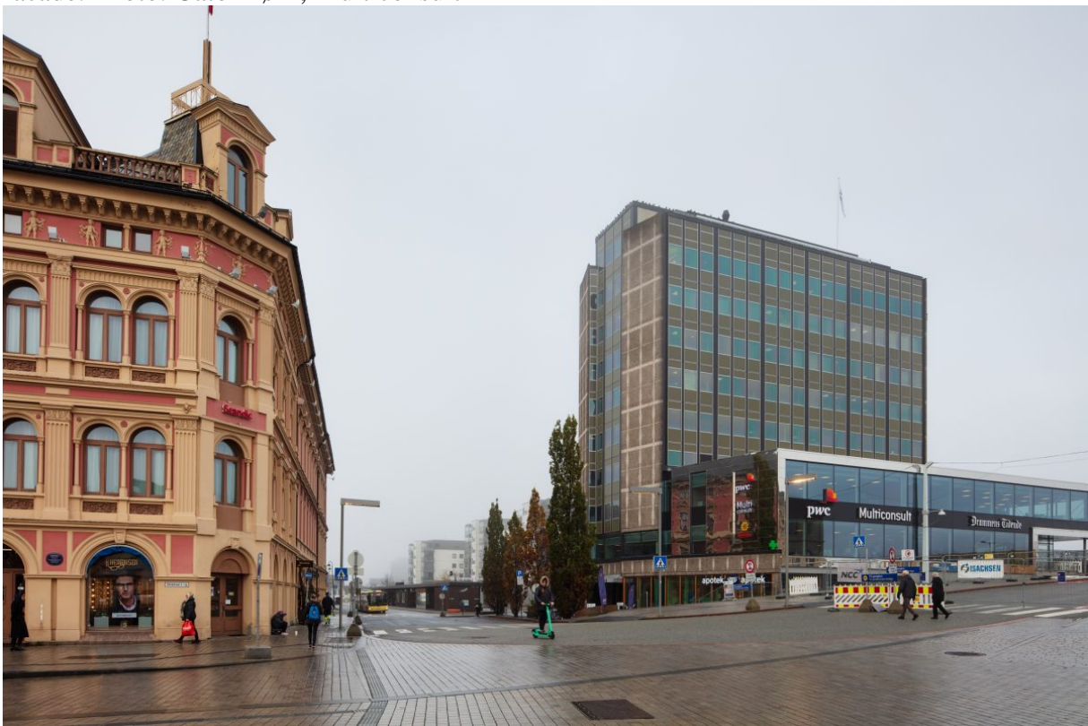
At Strømsø Square in Drammen, the old Sparebank building from 1962 has received new facade panels with integrated solar panels. The building was designed by the Nilsen and Grenager architect company and originally had green glass panels under the windows. There
