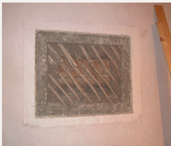
This building, which looks like an ordinary stone building has a timber core on the ground floor. The log wall is hidden behind a rendered facade. Inside the entrance area the wall has been reinforced with slanting hazel wood twigs. On the left is the “peephole” where you can glimpse the log wall on the inside. Oslo. Photograph: M. Boro © Riksantikvaren
