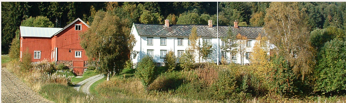
Trønderlag farmhouses, known as trønderlâne are very long and narrow. They are normally made up of several log cores side by side.
