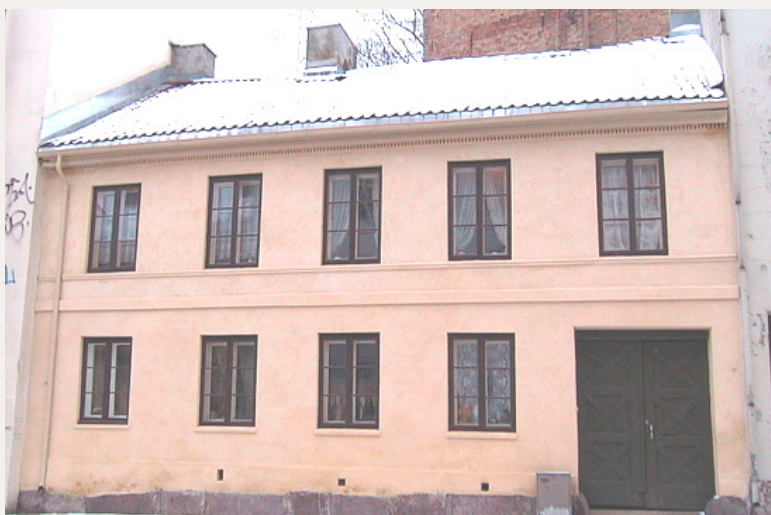
This building, which looks like an ordinary stone building has a timber core on the ground floor. The log wall is hidden behind a rendered facade. Inside the entrance area the wall has been reinforced with slanting hazel wood twigs. On the left is the “peephole” where you can glimpse the log wall on the inside. Oslo. Photograph: M. Boro © Riksantikvaren
